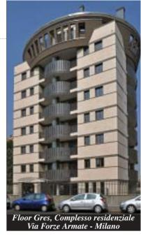
The Marazzi tiles that make up the ventilated façade display the alluring design of the black SistemA crystallized porcelain stoneware, an Ecolabel and Leed-certified, patented product made with over 40% recycled material, combined with building technology which allows for significant energy savings.
