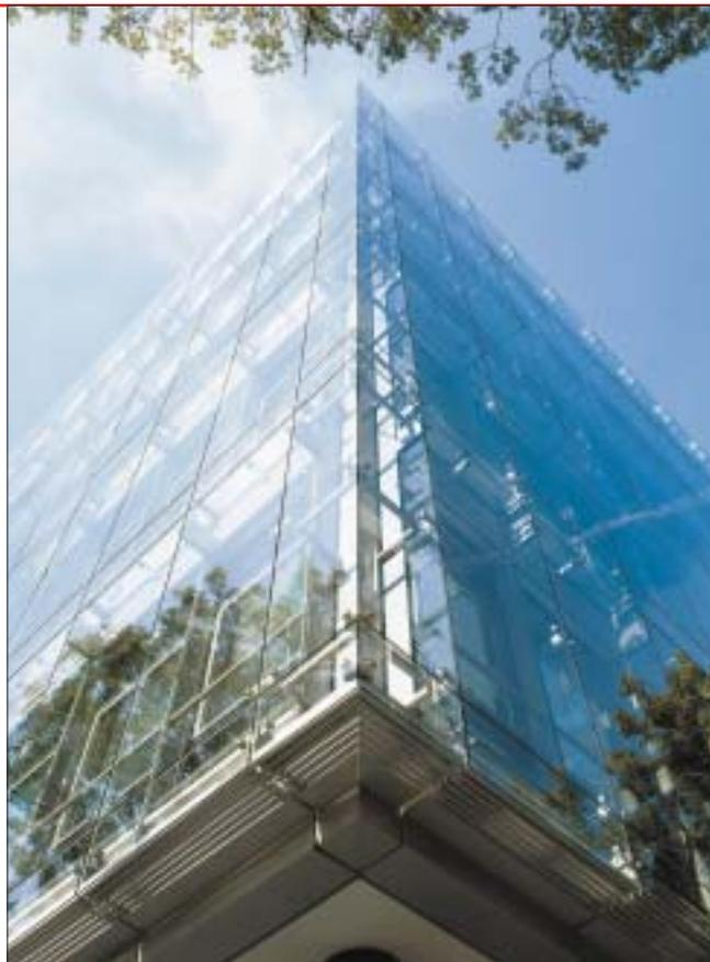
*solar control and enhanced thermal insulation. They reduce greatly solar gain and thermal heat losses. All products must be assembled into an insulating glass unit, with the coating facing the cavity of the unit.*
